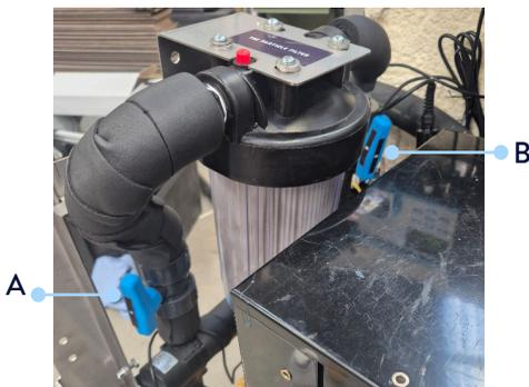
The isolation valves can be difficult to see, put your hand on the pipe to the left/right of the filter and follow this around until you get the valve.
